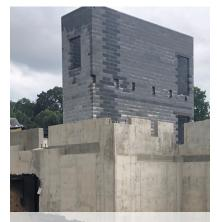
As seen in these photos, block stairtowers have been raised and steel bearing plates installed for structural steel to begin swinging over the jobsite.
